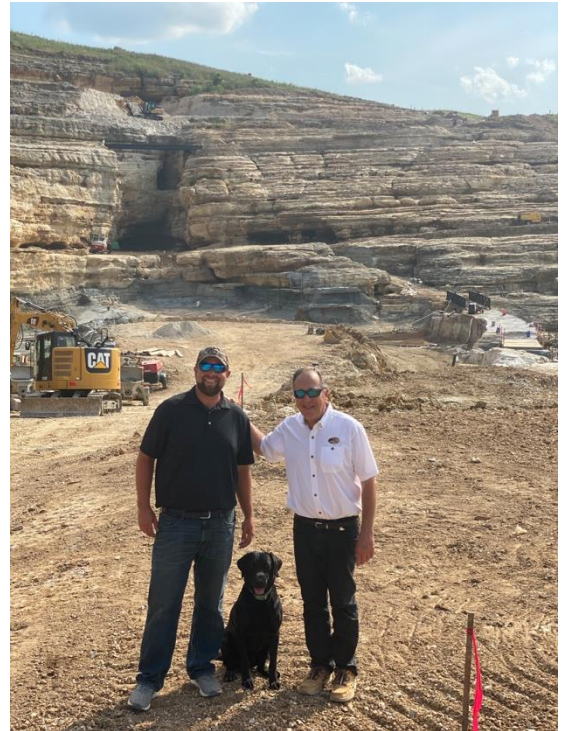
Johnny Morris, son JP and their buddy Roscoe during construction of the signature 19 th hole, envisioned by father and son at Payne's Valley.
